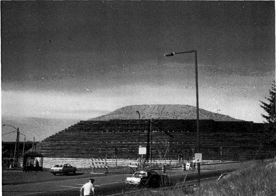
*View of the 12.6 m high Rainier Ave. wall supporting a more than 5 m high surcharge fill. This extensively instrumented structure is considered the highest geotextile-reinforced wall.*
