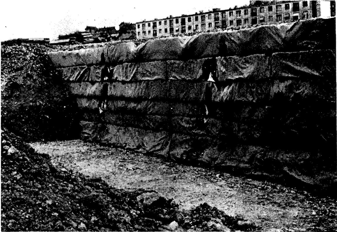
*First geotextile-reinforced wall, built in 1971 along freeway A15 in Rouen, France. This first wall was built using a poorly draining cohesive soil as backfill material.*
