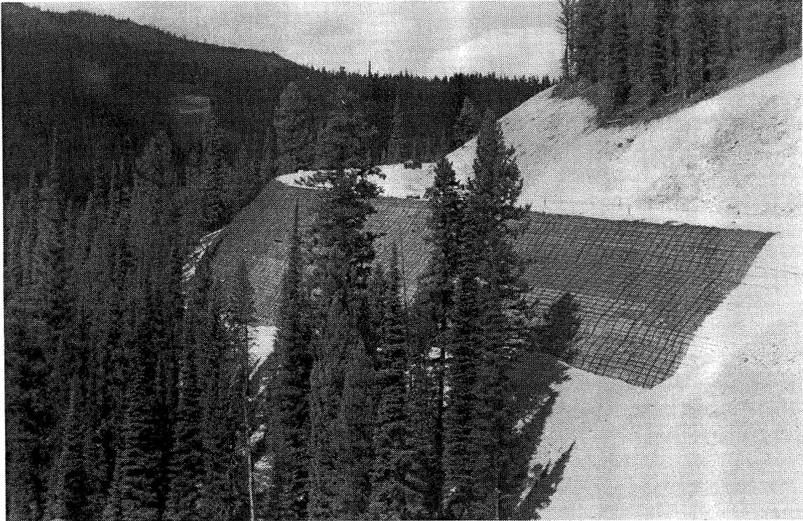
*View of a 15.3 m high geotextile-reinforced slope built using high strength geotextiles and decomposed granite as backfill material.*
