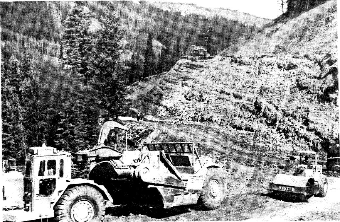
*Figure 5.5 - Rock shear key under construction*
