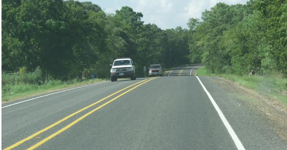
Figure 4.25 Example picture of the field performance of the test section stabilized using GG 1 at FM 1774
