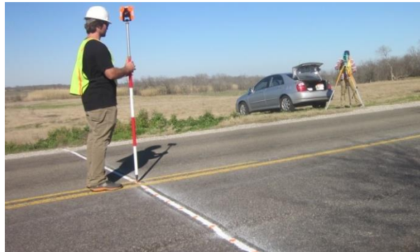
Figure 4.6 Using total station and prism to monitor vertical deformation of the marked transverse sections
