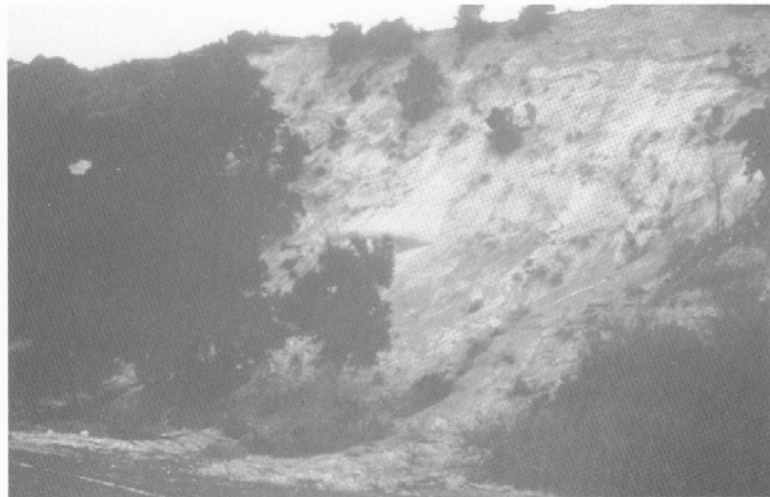
Figure 15. Rockslide along Santa Susana Pass Road, near the pass.
