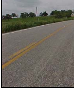
Geogrid Section 1: No longitudinal cracks
