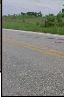
Control Section: Longitudinal cracks
