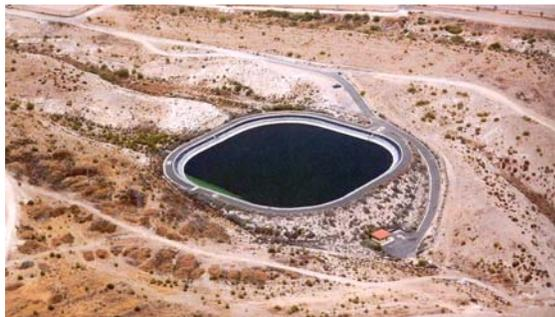
Figure 1. Reservoir of “San Isidro” waterproofed with HDPE.
