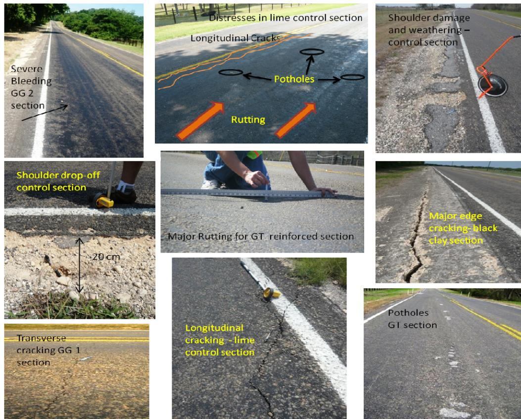
Figure 9. Overview of different distresses observed for various sections in FM 2
