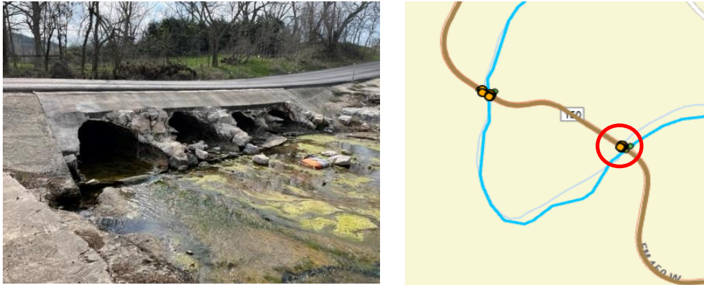
Figure 3.2. Low water crossing pipes and geographic location
