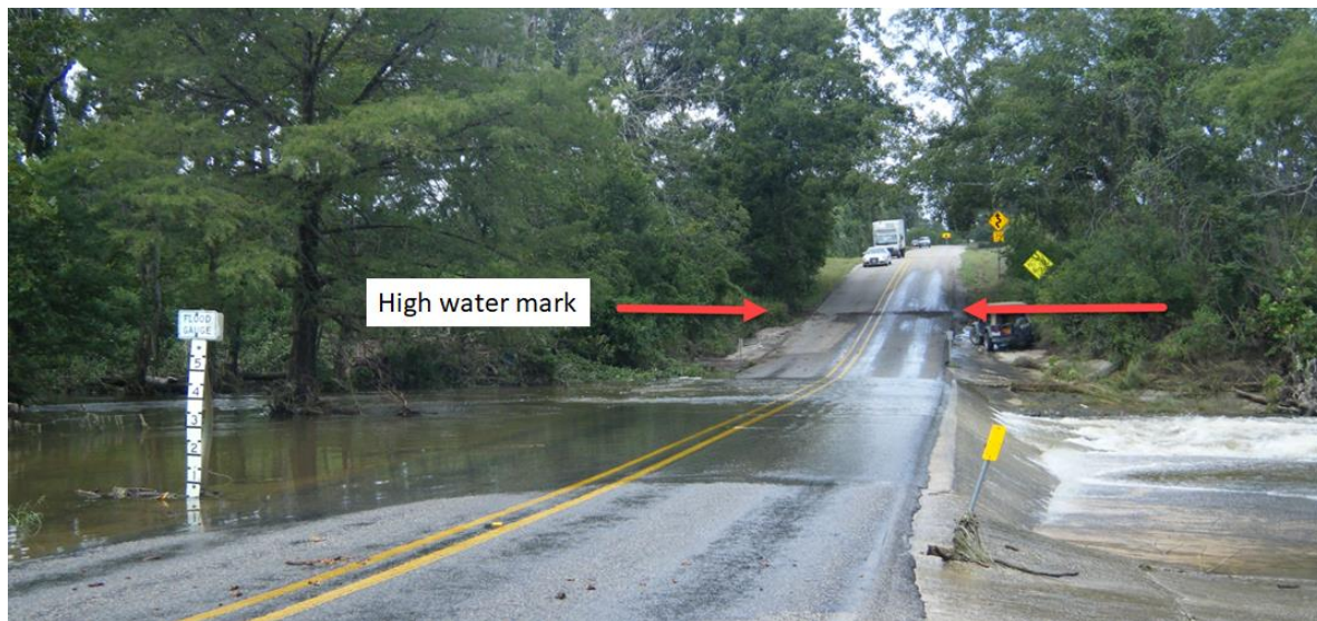
Figure 3.1. Low water crossing on FM 150 at Onion Creek near Driftwood, Texas showing the high water mark for a flood event inundating this road.
