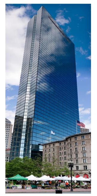
Boston's John Hancock Tower (241 m, 60 floors) was originally vibrating excessively at wind speeds > 45mph and causing windows to fall (...became the "Plywood" palace!)
