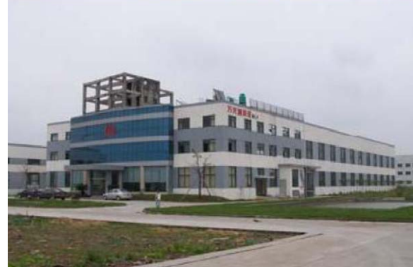
Fig. 27. Two-stage solar desiccant cooling system installed in Jiangsu, China.
