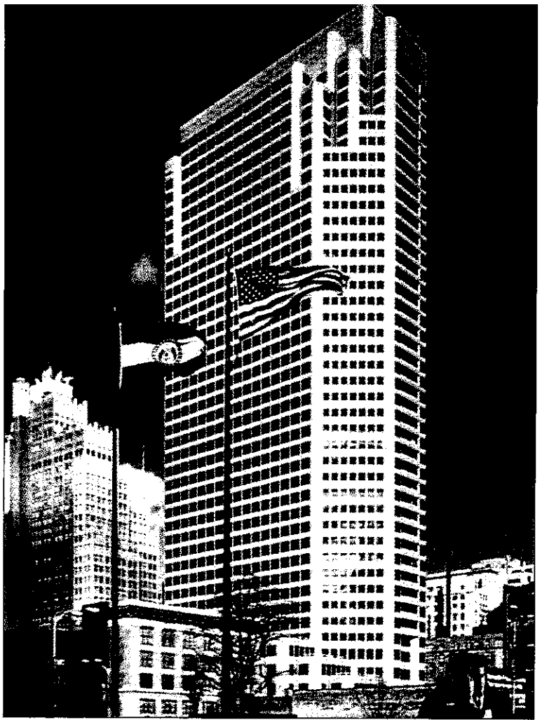
Plate 8 Southwestern Bell Telephone Company in St. Louis, USA. Architects: Hellmuth, Obata & Kassabaum, USA. M/E Engineers: William Tao & Associates, USA.
