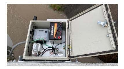
Figure 3.2.2. Equipment housed in the gauge enclosure
